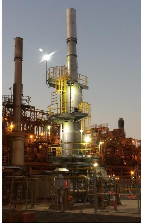
The new unit (left) has 4 times the capacity of the old unit. The old unit will now be on standby, allowing the plant to have a thermal oxidiser operating and destroying some of the site's odour at all times.
