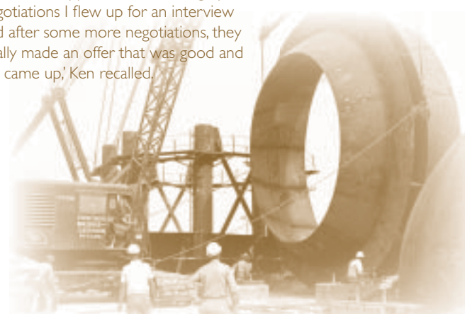
▼ Precipitator tank erection. Photograph by Burton S. Block.
