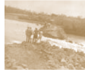
▲ Water breaking through the first attempt to build the Red Mud Dam. Image courtesy Frank Bowen.
