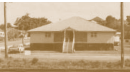
▲ (Top) The men's hostel at 2 Roseberry Street before renovations. (Bottom) The men's hostel at 2 Roseberry Street after renovations.
