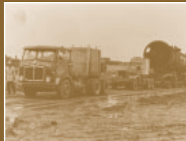
Pressure vessel being transported through Gladstone and being put in place at QAL, 1965. (including cover)
